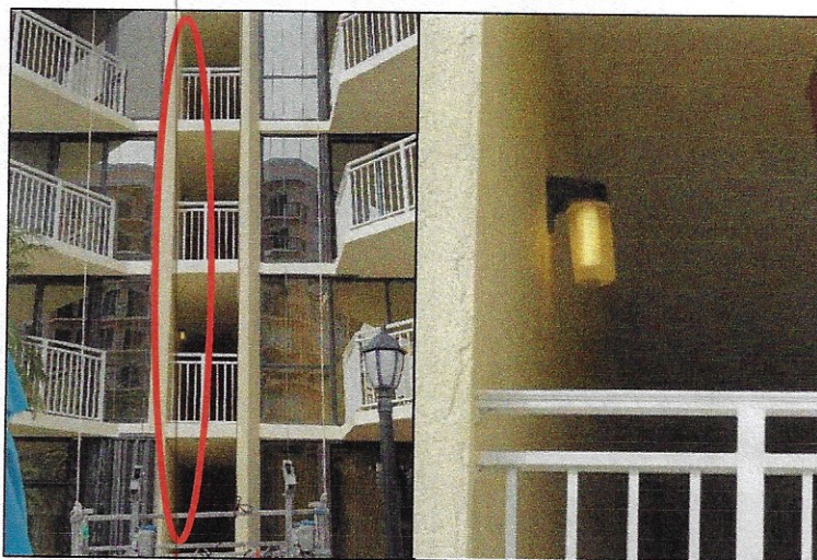
Figure 7: Photos of the existing wall mounted fixtures in the south facing hallway, circled in red and a close-up of the existing wall mounted fixture.
