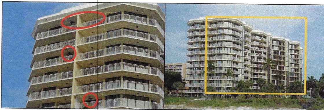
Figure 6: Photos of the existing ceiling fan light kits that are to be removed, circled in red, and the south facing side of the building with the existing ceiling mounted balcony fixtures, outlined in yellow.
