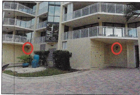
Figure 8: Photo of the existing wall mounted lantern style fixtures near the service entrance, circled in red.
